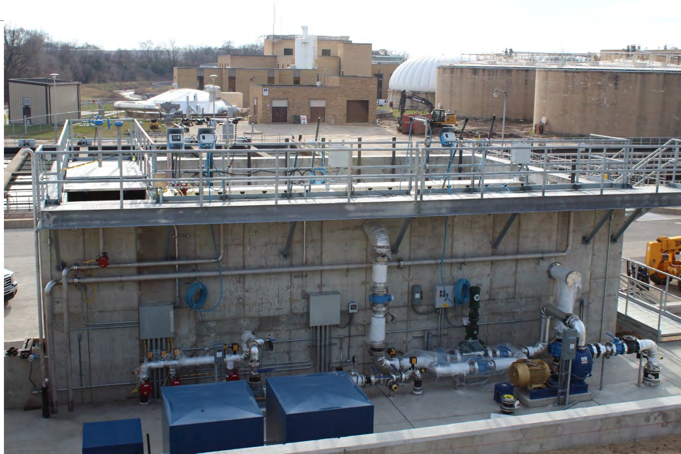
AASI breaks ground at FRSA for first AquaNereda® System in North America
