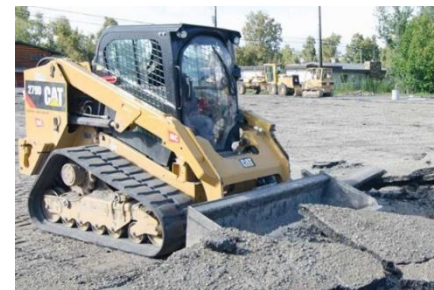
PAVEMENT REMOVAL
