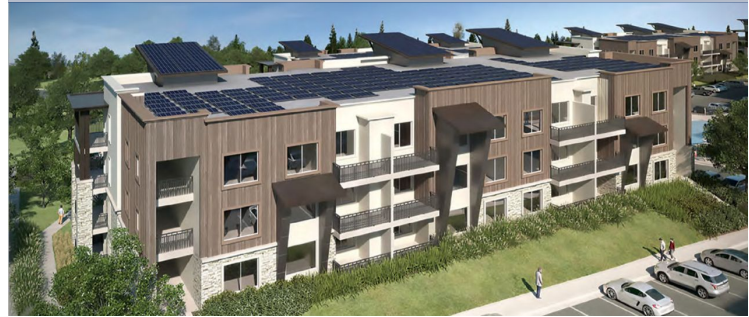
SOLEIL LOFTS, POWERED BY SOLAR & STORAGE Herriman, Utah
