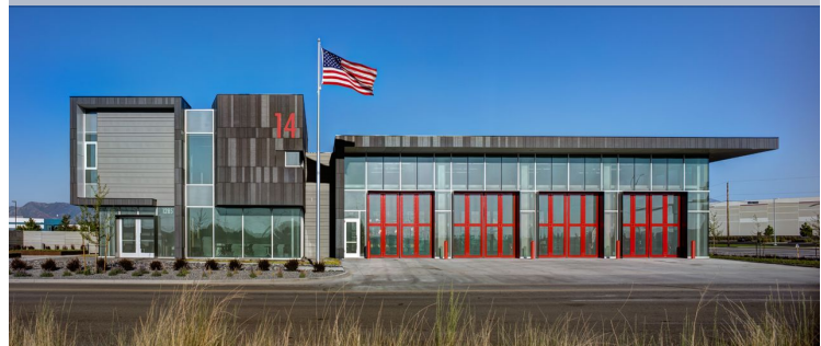
FIRST NET-ZERO FIRE STATION Salt Lake City, Utah
